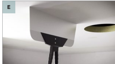
Check joints and center of panels.
