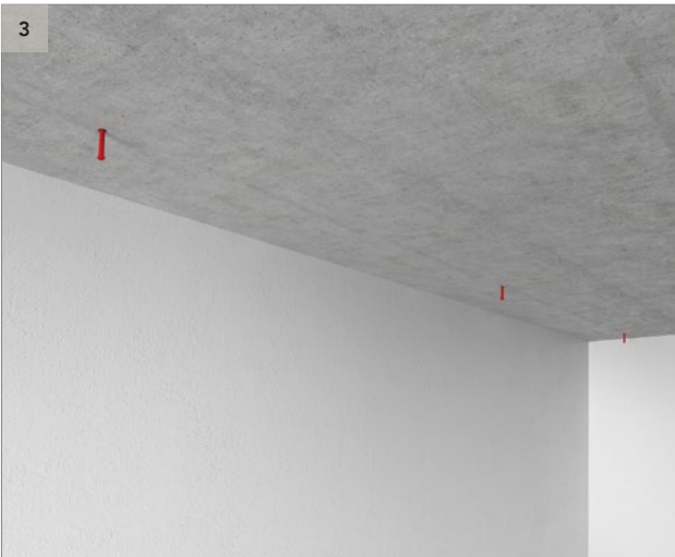
Use fixings that are appropriate for the soffit.
