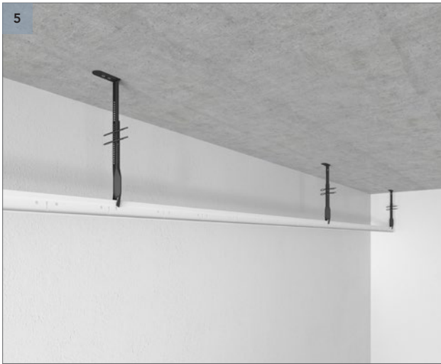
Attach T24 ECR main runners by bottom parts of nonius hangers to the top parts of nonius hangers and lock with two locking pins.
