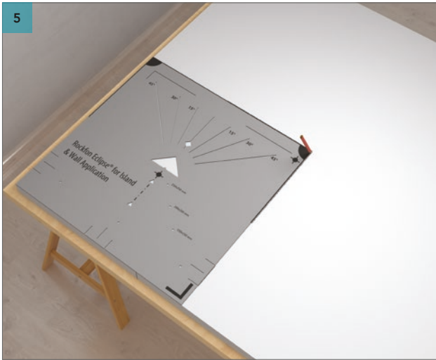
Position the marking tool in the lower left corner on the back side of the Rockfon Eclipse Wall panel. Mark with a pencil the centre lines, using the upper right corner of the marking tool, and the position of the distance holder. See 5 - Result.
