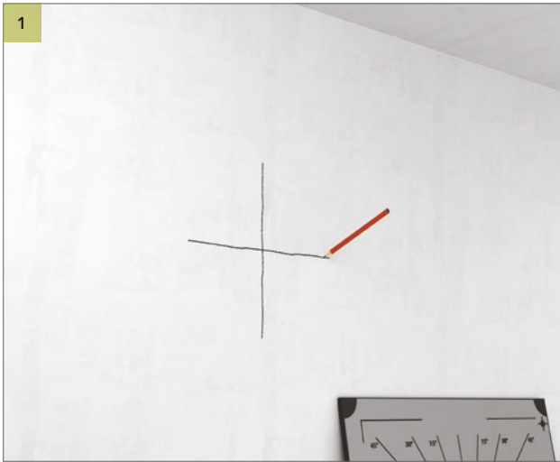
Mark a cross on the wall to indicate where you intend to fix the centre of your Rockfon Eclipse Wall panel. Make sure the upper leg of the cross is +/- 30 cm.
