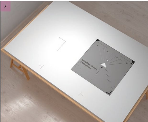
Mark the line where the panel fixing profile must be inserted. Do this to both the right and left side of the wall panel. See 7 - Result.
