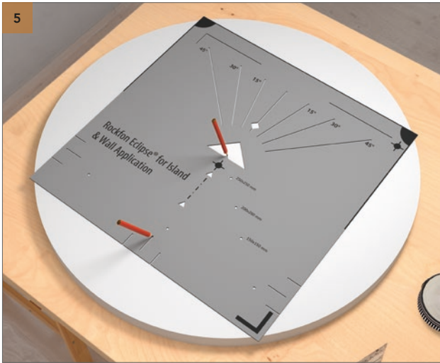
Position the marking tool on the backside of the wall panel and mark with a pencil the base of the triangle and the position of the distance holder. See 5 - Result.
