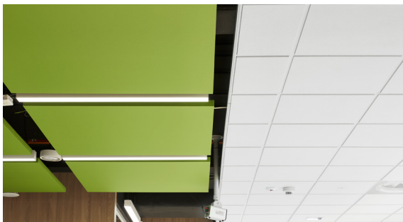
Architect Aleksandra Czubaszek-Situch from Kuryłowicz & Associates Products Rockfon Eclipse® Colour, Rockfon® Koral™, Rockfon® MediCare® Plus
