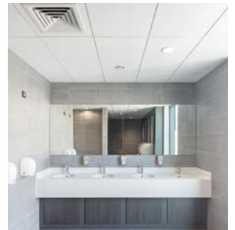
Toilet & Locker room / 32
